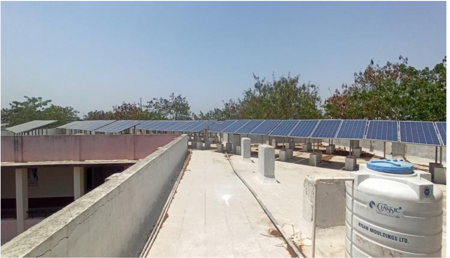
Solar Installation at School of Commerce
