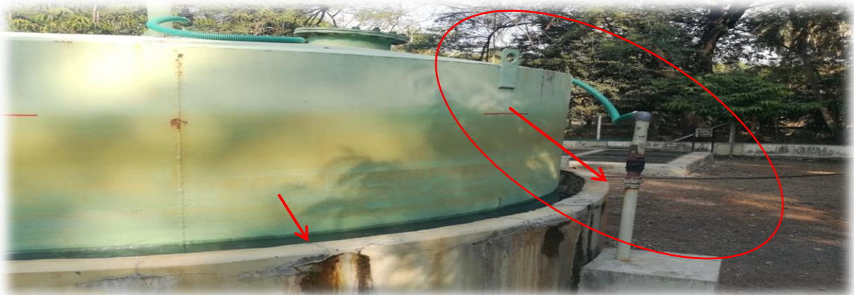
Picture 16: Floating Dome
