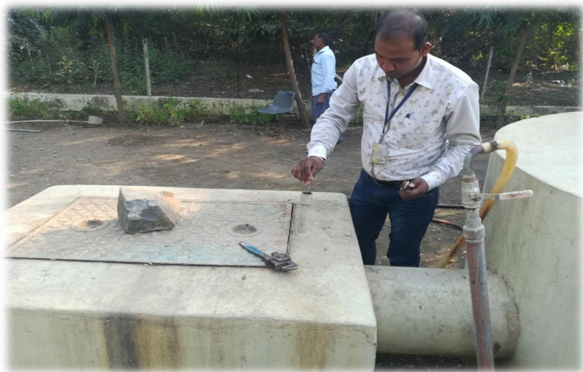
Picture 12: Inspection Chamber-I
